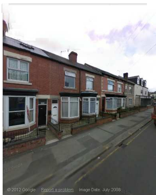
Photograph 1 Residential Properties (Wolsey Road) immediately opposite the extension
